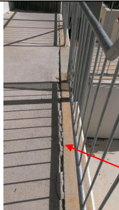
29. Item 31 – concrete spalling along edge
