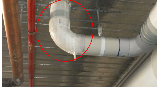
19. Item 16 – leak through joint above
