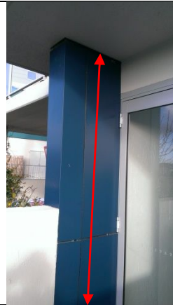
42. Item 126 – failed cladding
