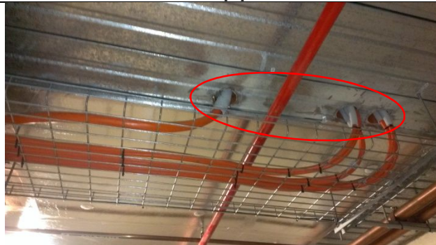
13. Item 5 – leak around pipe
