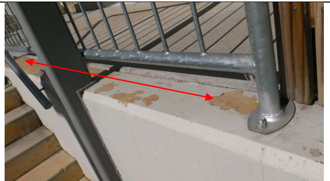
28. Item 30 – paint failure
