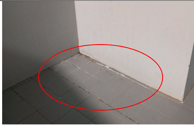
25. Item 26 tile failure to East BBQ area
