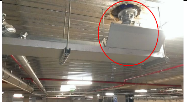
24. Item 21 – leaks through pipe penetrations
