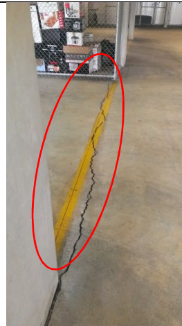
16. Item 9 – floor crack to be sealed
