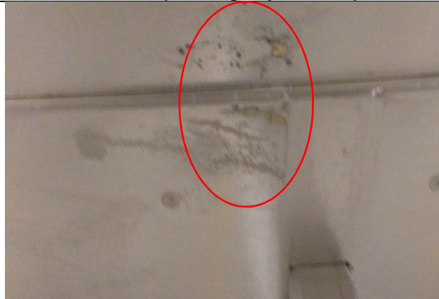
11. Item 3 – leak through insulation adj space 14
