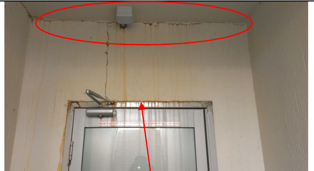
28. Item 30 – paint failure
