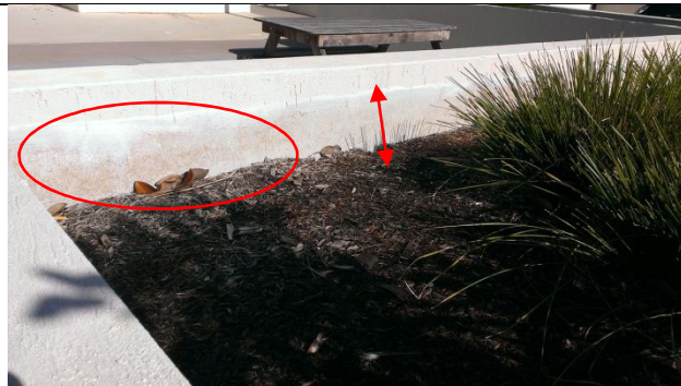
27. Item 29 – soil levels dropped – membrane exposed
