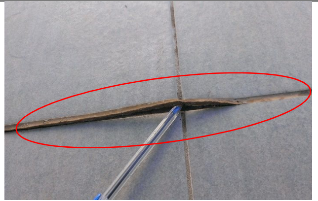
26. Item 27 – sealant failure to E BBQ area
