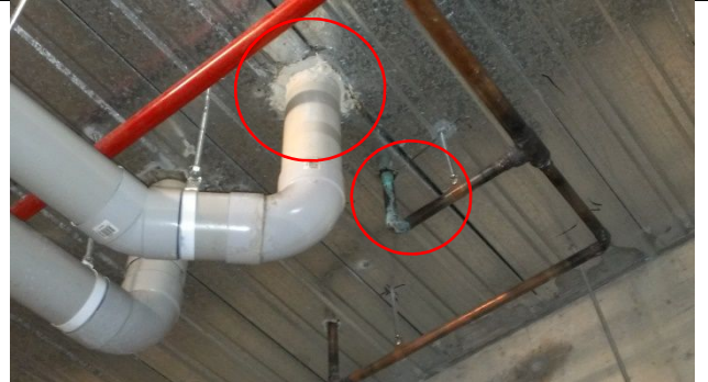
14. Item 6 – leak around pipes
