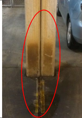
19. Item 16 – leak through joint above
