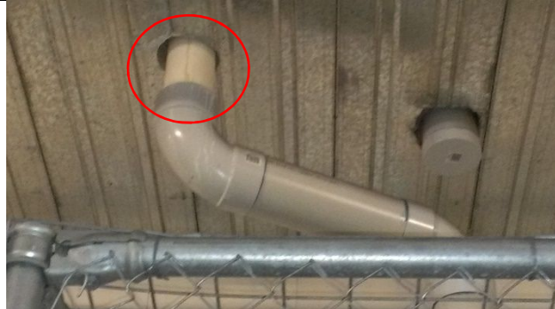
13. Item 5 – leak around pipe
