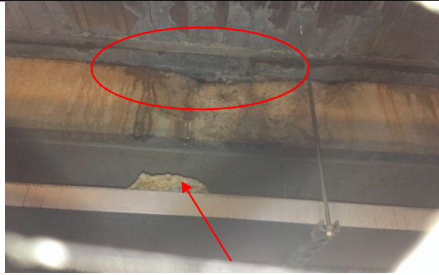
1. Item B – spalling concrete
