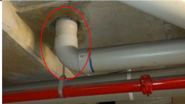
23. Item 20 – leak through pipe penetration
