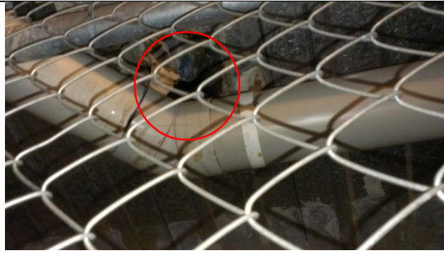
17. Item 12 – leak around redundant penetration
