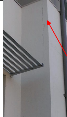
2. Item D – typical render cracking
