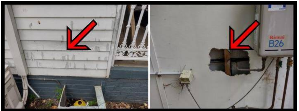
The condition of the walls is generally fair. Cladding is damaged, repairs and maintenance will be required. Paint deterioration was present to external surfaces. Maintenance and/or repairs will be required.
