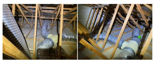
**Roof Frame Type** The roof frame is a truss timber frame.
